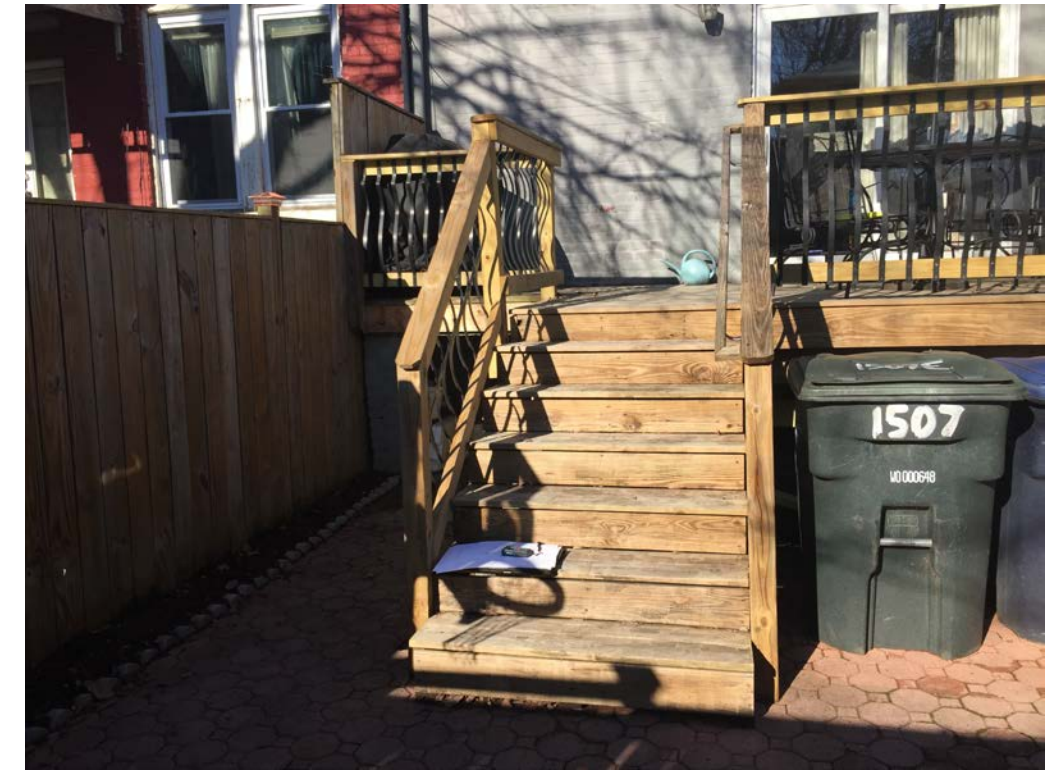
EXISTING DECK & STEPS TO GRADE
