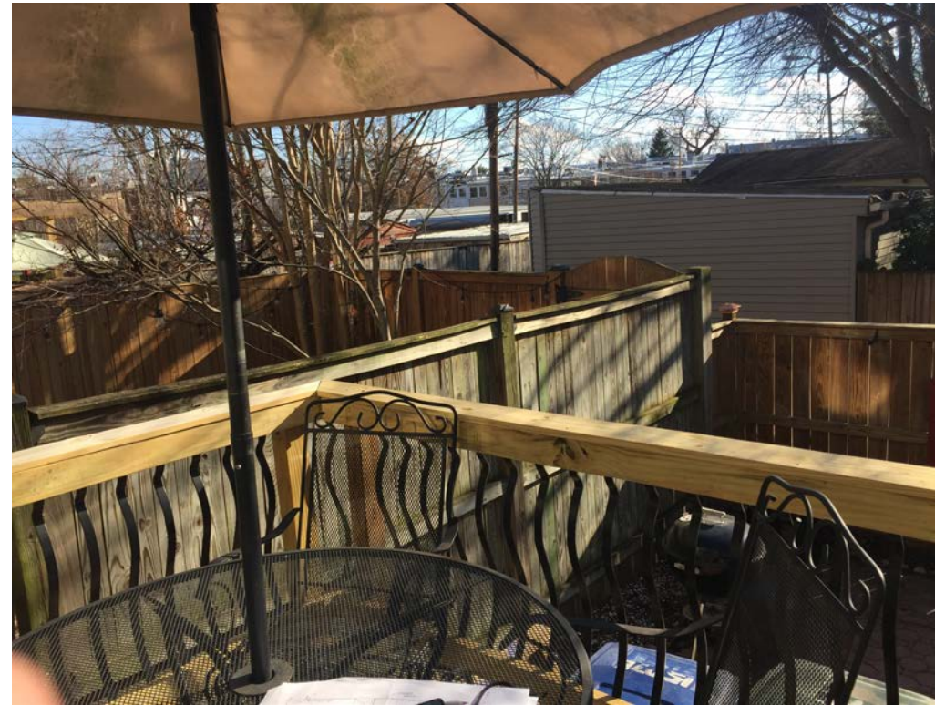
VIEW FROM EXISTING DECK, LOOKING EAST
